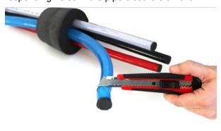
Cut off the hose ends in order to remove the punch residue.
