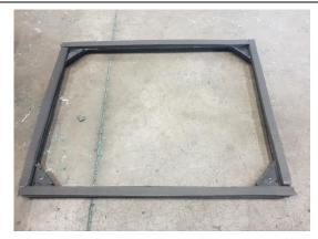
Set the original lid frame (including neoprene seal) in place on top of the collar and use the existing holes to drill some pilot holes on the top of the riser set. Secure the lid frame in place using the original NO.14  $\times$  1.5" screws.
