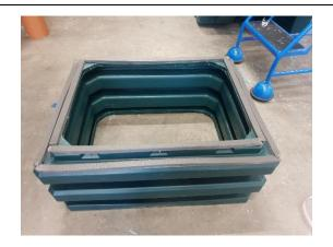
Set the 450mm by 600mm riser in place on top of the tank where the lid frame used to be located
