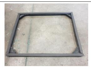
Set the original lid frame (including neoprene seal) in place on top of the collar and use the existing holes to drill some pilot holes on the top of the riser Secure the lid frame in place using the original NO.14  $\times$  1.5" screws.
