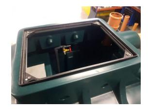
Check that the riser has been trimmed and confirm the 5mm pilot holes have been drilled out. If not, use a 5mm drill bit and use the drill spots on the bottom of the tool (3 on each of the long side and 2 on each of the ends)
